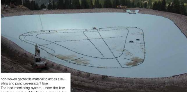
non-woven geotextile material to act as a levelling and puncture-resistant layer.
