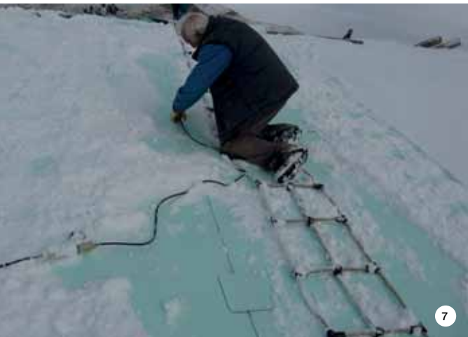
PHOTOS 5 and 6. Installing MAPEPLAN T WT onto the sides and bottom of the water reservoir.
