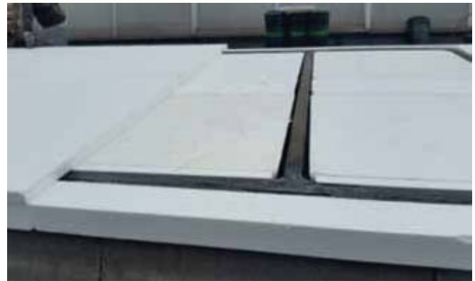
APPLICATION OF EPS INSULATING PANELS
