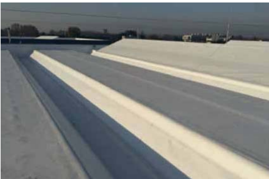
THE ROOF AFTER COMPLETION OF THE WORKS
