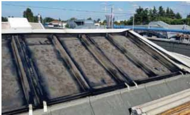
APPLICATION OF POLYVAP RADONSHIELD VAPOUR BARRIER
