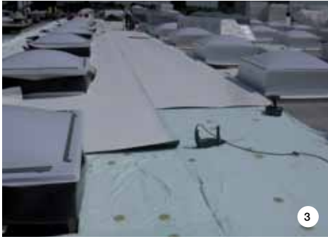
PHOTO 3. Laying and fastening MAPEPLAN T M membrane in place.
