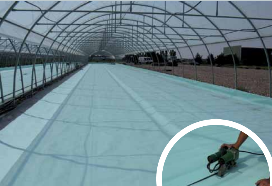
The water tanks were waterproofed using MAPEPLAN T WT.
