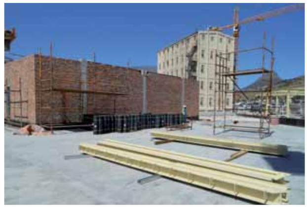
Waterproofing work on one of the terraces in the Silo District.
