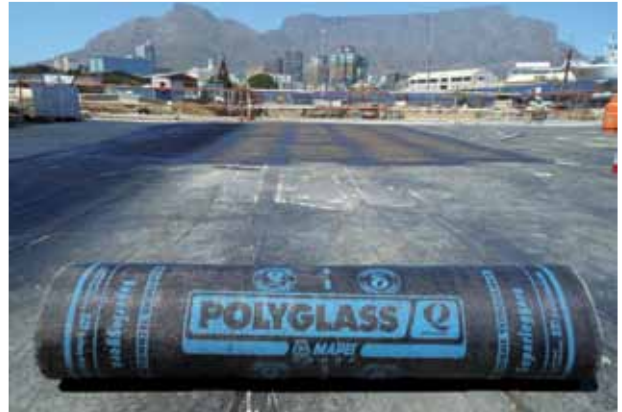
Application of a REOXTHENE® membrane in one of the silos.
