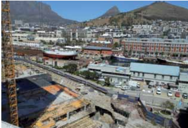
The foundations for Silo 1 from above.
