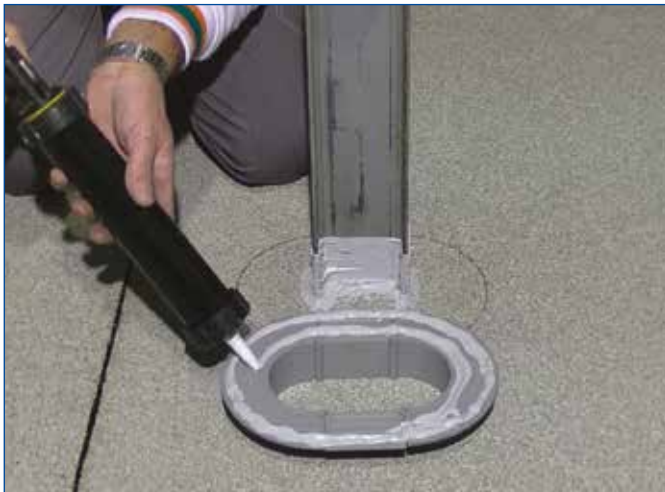
FIGURE 4 - Application of the POLYSEALANT CARTRIDGE adhesive sealant
