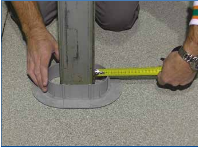
FIGURE 3 - Positioning of the formwork
