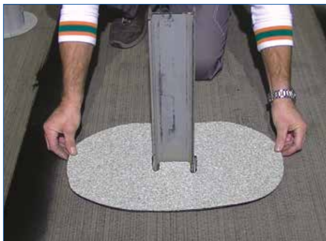
FIGURE 7 - Application of patch of mineral membrane
