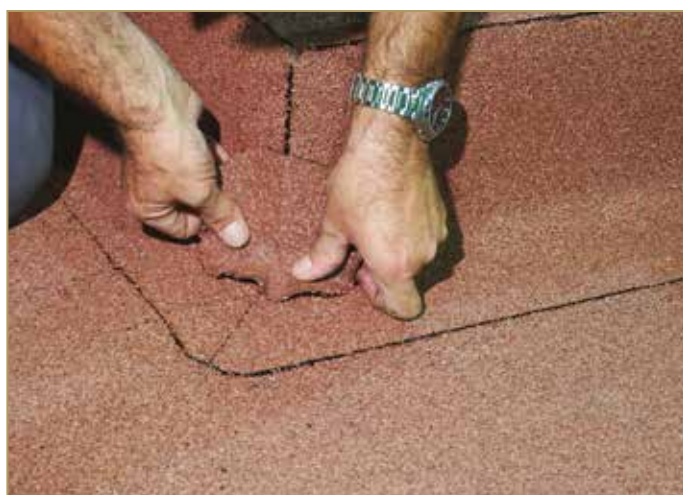
Figure 9.66: Preparing the closing membrane patch
