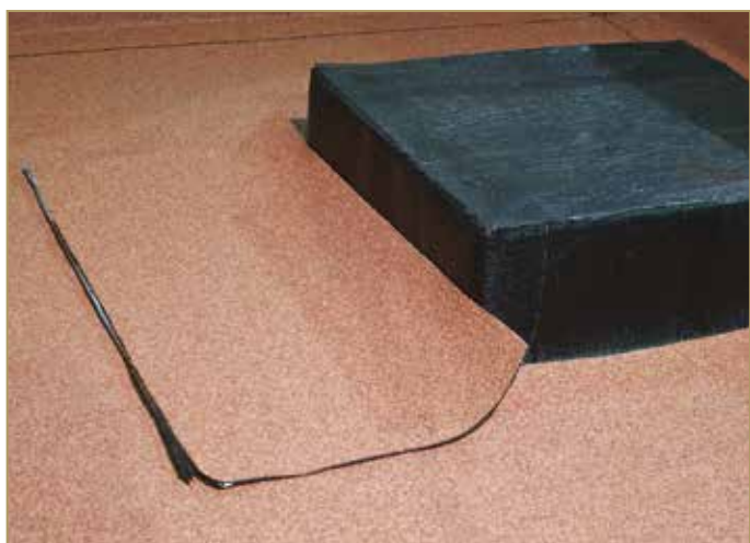
Figure 9.52: Preparing the vertical up-turn of the second waterproof layer with slate chipping finish
