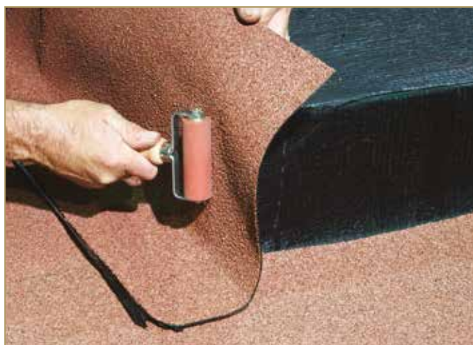
Figure 9.53: Gluing and rolling the vertical up-turn
