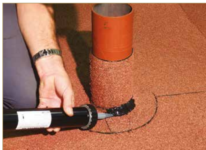
Figure 9.104: Sealing the tube base connection with POLYDETAIL MS
