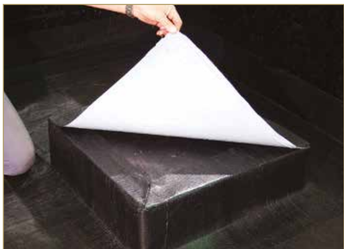
Figure 9.50: Preparing the top of the protruding structure
