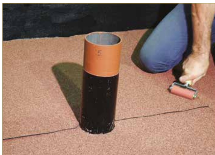
Figure 9.93: Rolling the overlaps
