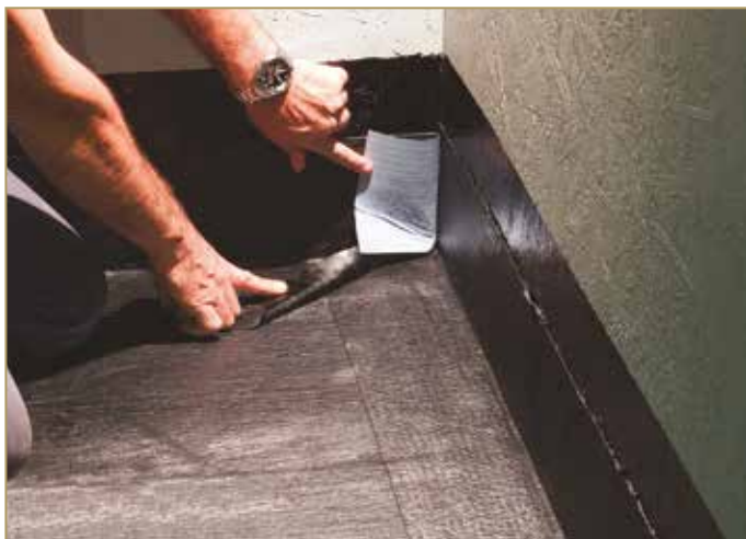
Figure 9.1: Preparation of the internal corner
