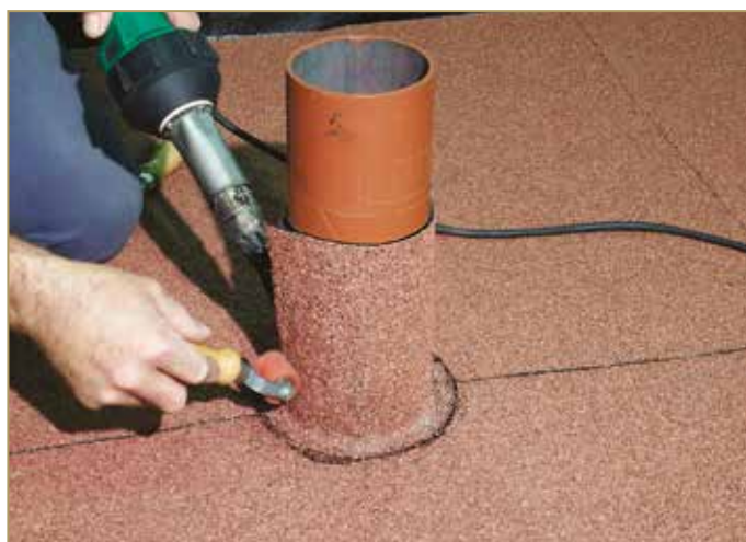
Figure 9.99: Welding the overlap on the vertical tube
