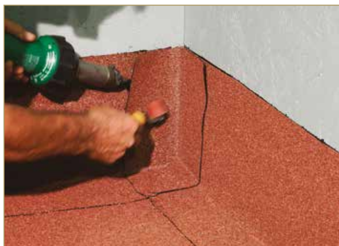
Figure 9.26: Welding the patch on the vertical wall
