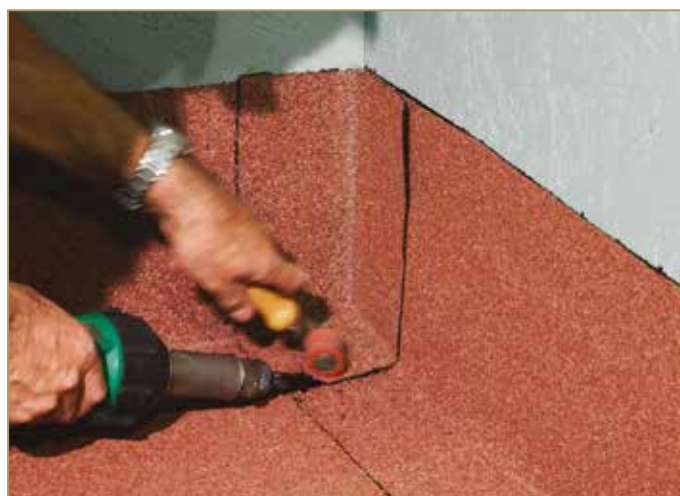
Figure 9.28: Hermetically closing and welding the corner
