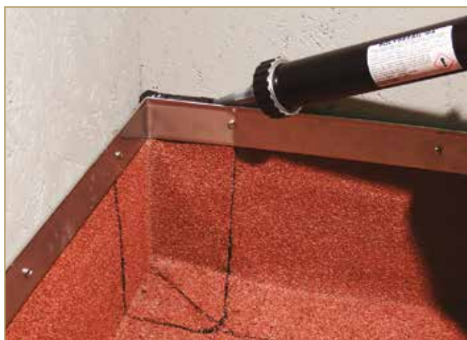
Figure 9.34: Sealing using POLYDETAIL MS
