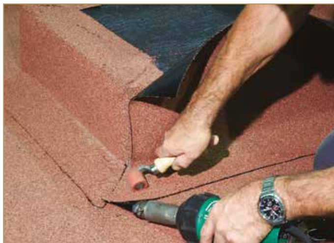
Figure 9.61: Welding the overlap on the flat surface
