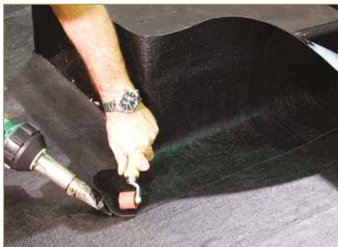
Figure 9.37: Welding the overlap on the flat surface
