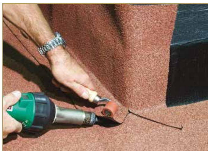
Figure 9.55: Welding the overlap on the flat surface
