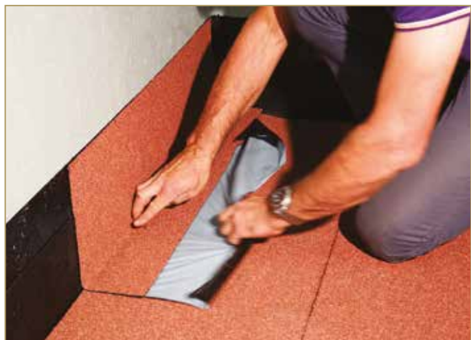
Figure 9.17: Removing the protective film
