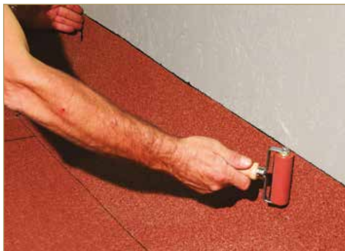
Figure 9.20: Rolling the vertical detail
