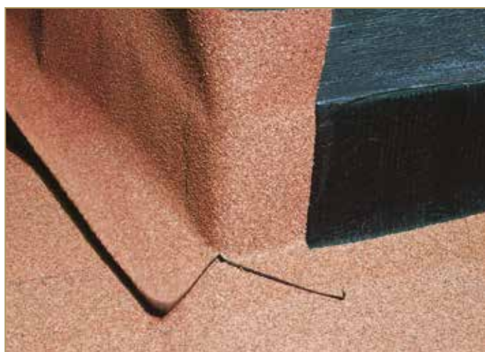
Figure 9.54: Cutting at 45° and folding the up-turn on the corner
