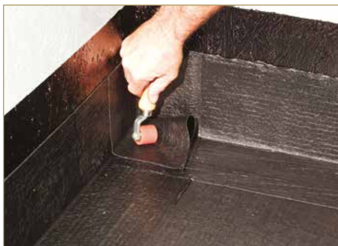
Figure 9.10: Horizontal gluing and rolling
