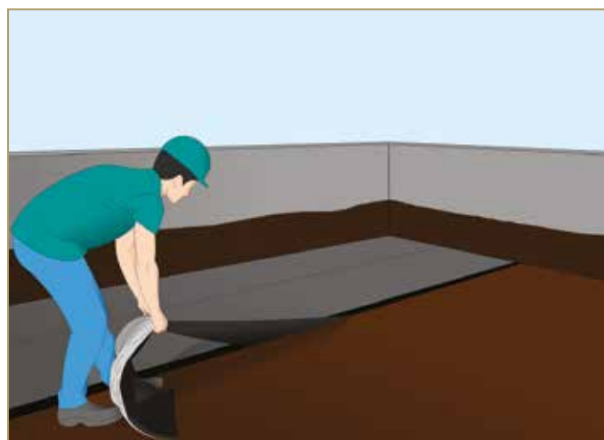
Figura 7.10: Remove part of the release mono-silicone protective film on the bottom side, to adhere the first half of the membrane
