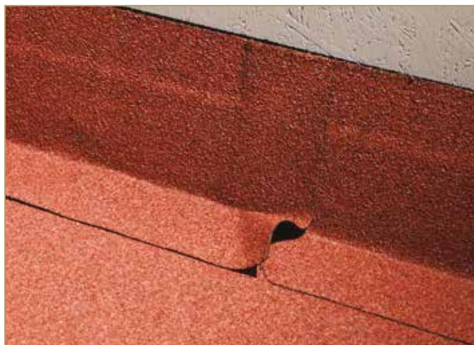
Figure 9.30: Overlap of two adjacent vertical up-turn
