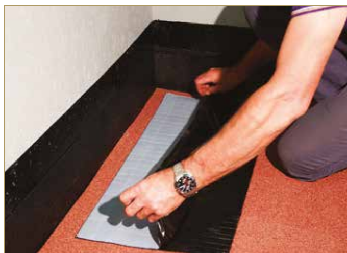
Figure 9.14: Partially removing the protective film
