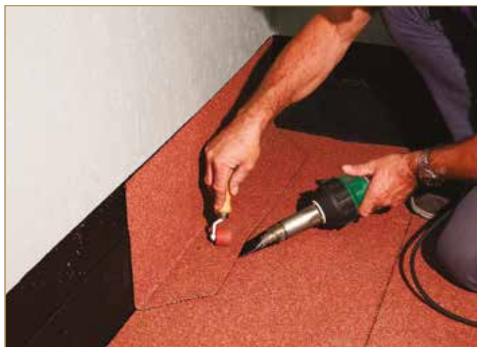
Figure 9.18: Welding the overlap on the flat surface
