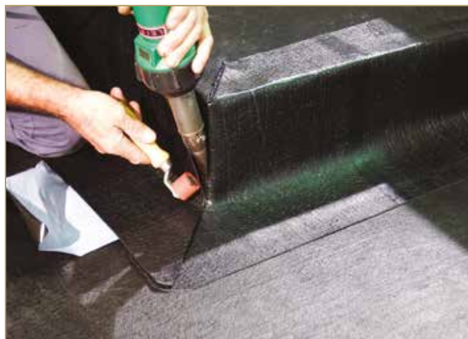
Figure 9.43: Up-turn at vertical welding
