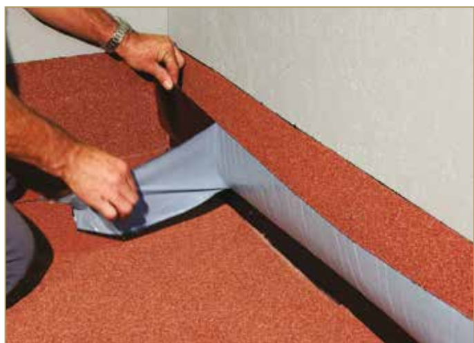
Figure 9.21: Total removal of the release film
