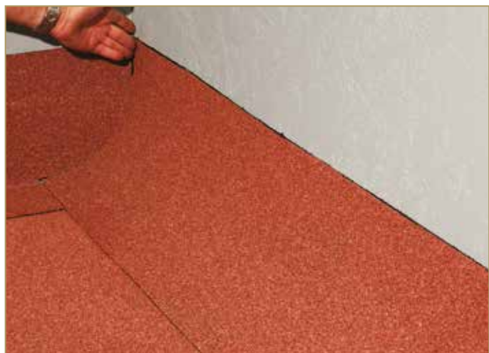
Figure 9.19: Preparing the vertical up-turn on the adjacent wall
