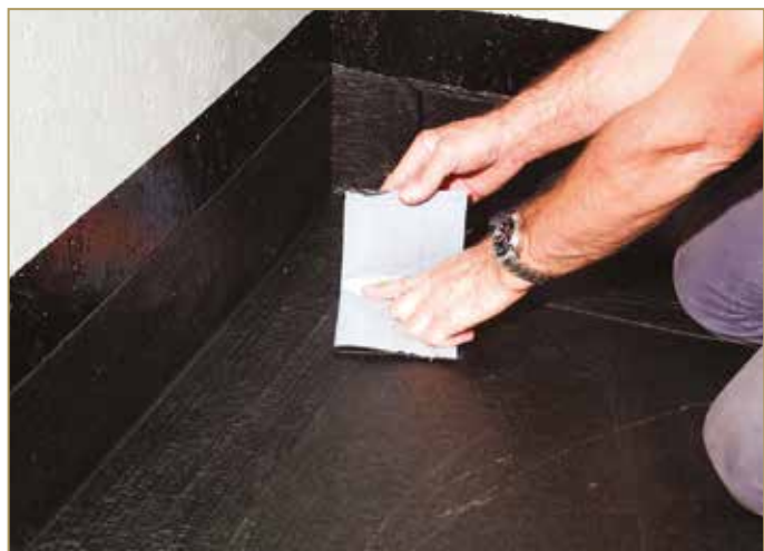
Figure 9.5: Folding the patch of membrane into 4 parts
