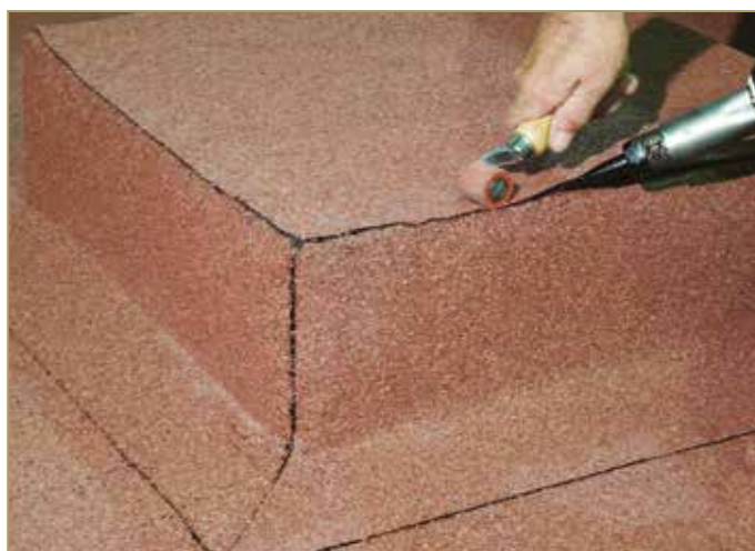
Figure 9.65: Welding the upper edge
