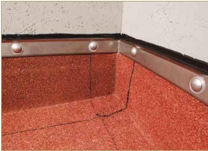
Figure 9.35: Completed internal corner with profile and studs
