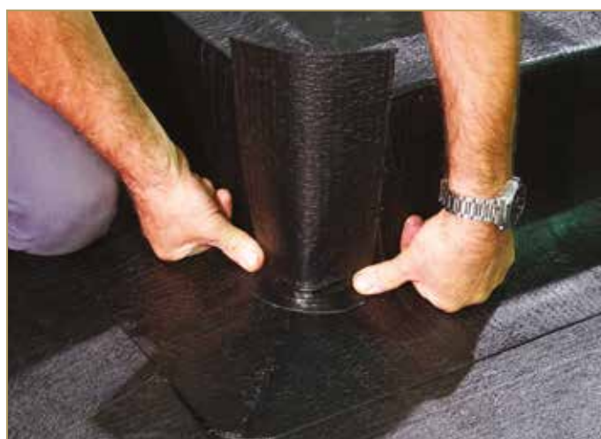
Figure 9.47: Positioning and gluing the closing patch
