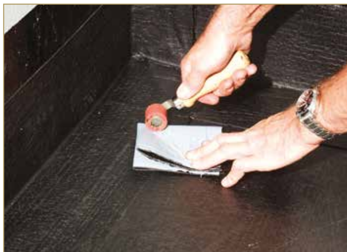
Figure 9.6: Rolling to mark the 4 corner portions
