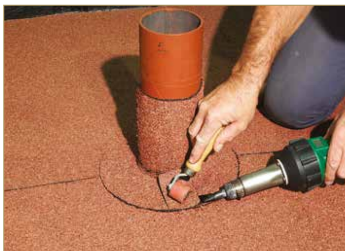
Figure 9.103: Closing weld of the patch cut
