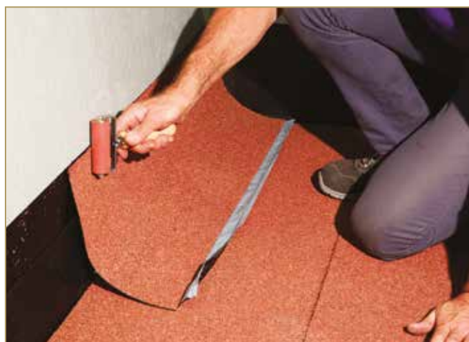
Figure 9.16: Rolling the top part
