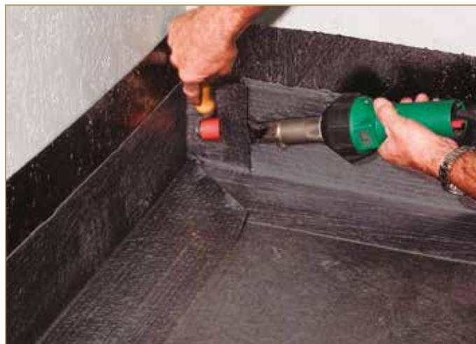
Figure 9.2: Up-turn vertical welding
