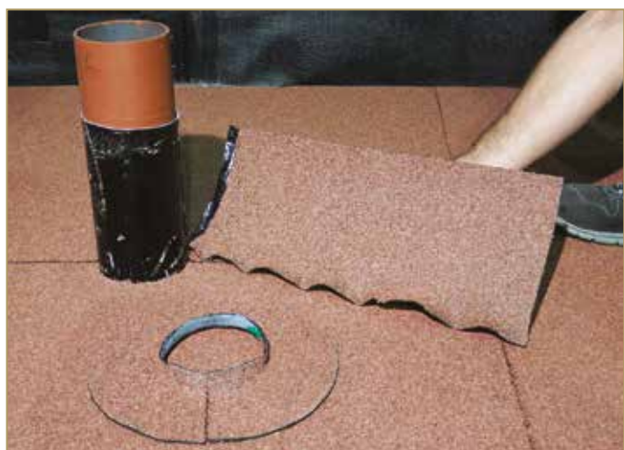
Figure 9.95: Preparing the elements to line the tube
