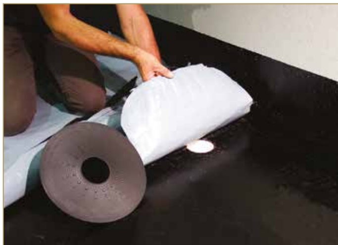
Figure 9.69: Preparing the membrane to place under the outlet flange for vapour barrier 50x50 cm
