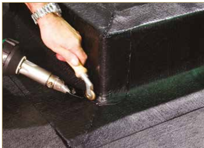
Figure 9.49: Welding the patch on the flat surface
