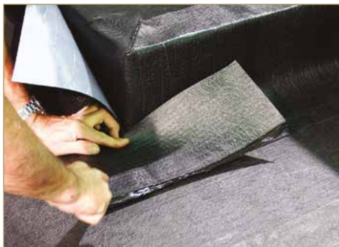
Figure 9.41: Cut at 45° of the overlapping part on the flat surface
