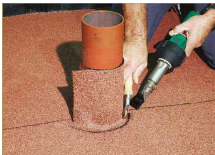
Figure 9.97: Welding and rolling the up-turn foot
