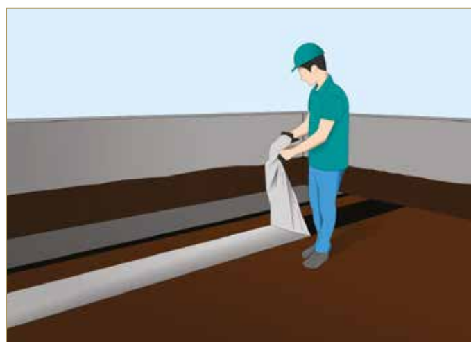
Figure 7.12: Remove the second half of the release mono-silicone protective film
