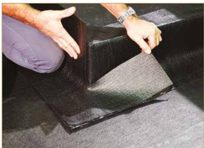
Figure 9.40: Making the part of vertical up-turn adjacent to the first one
