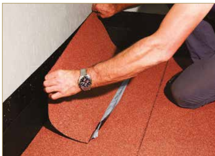
Figure 9.15: Positioning and gluing on the vertical up-turn
