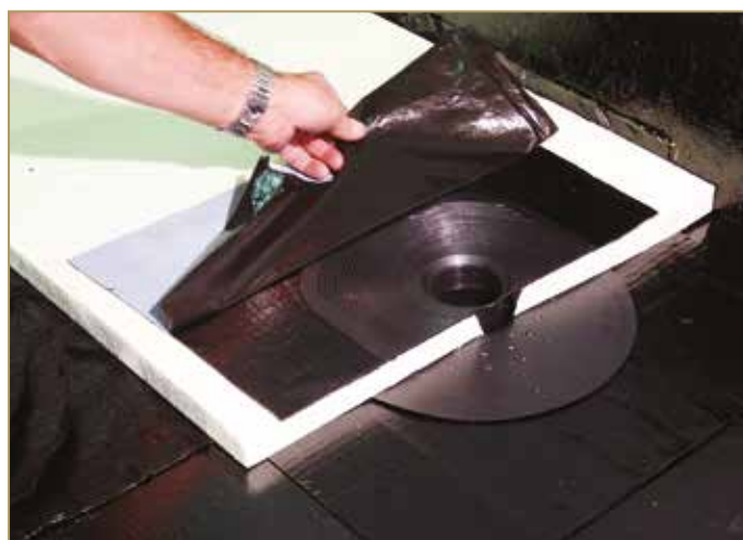
Figure 9.78: Removing the protective film
