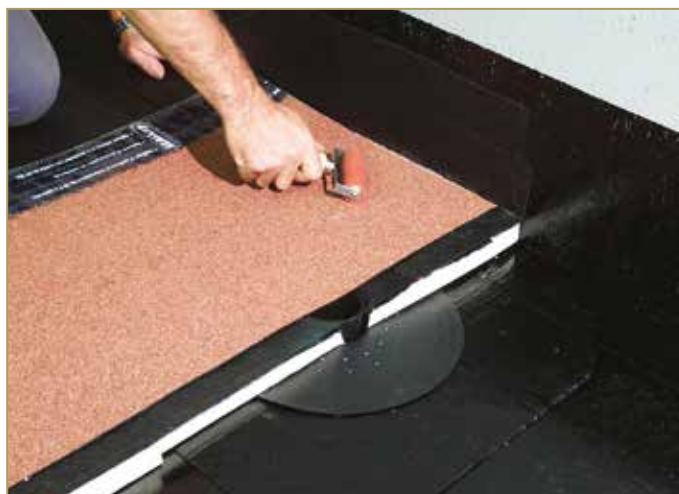
Figure 9.84: Rolling and gluing on the flat surface
