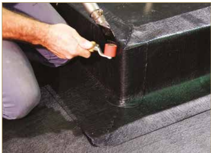
Figure 9.48: Welding the patch on the vertical wall
