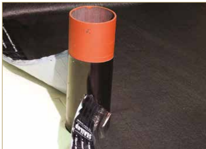
Figure 9.87: Positioning and cutting the first waterproof layer
