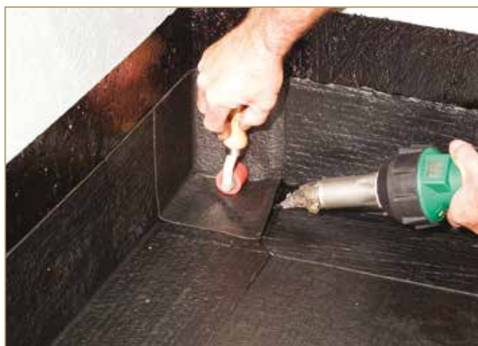
Figure 9.11: Hermetically closing and welding the corner
