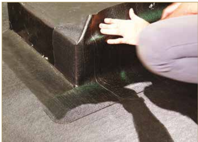
Figure 9.38: Folding the membrane on the upper edge
