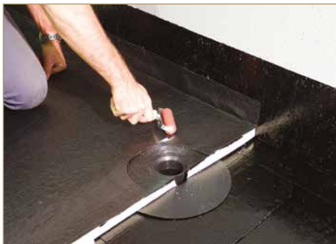
Figure 9.81: Membrane gluing and rolling
