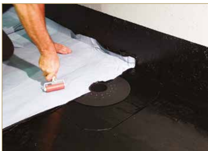
Figure 9.73: Positioning the ADESO vapour barrier and rolling
