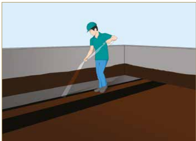
Figure 7.13: Remove the protective film on the side seldge of the adjacent membrane
