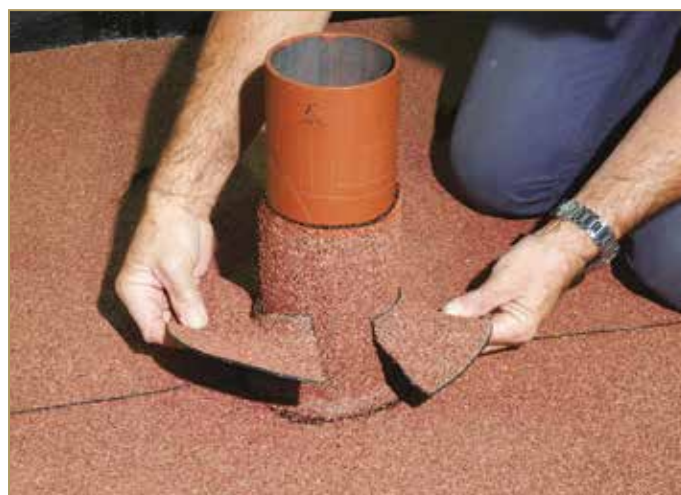
Figure 9.100: Positioning the covering patch
