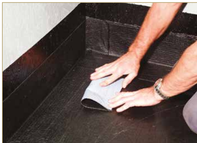
Figure 9.4: Cutting a 20x20 cm patch of membrane
