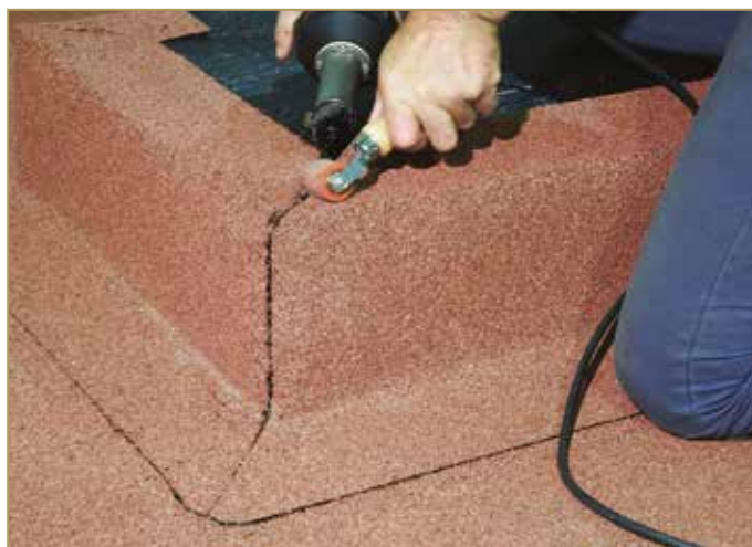
Figure 9.63: Welding the upper corner
