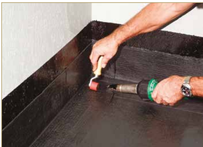
Figure 9.3: Flat welding
