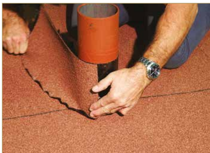
Figure 9.96: Gluing the vertical up-turn on the tube
