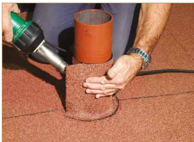
Figure 9.98: Welding the vertical part
