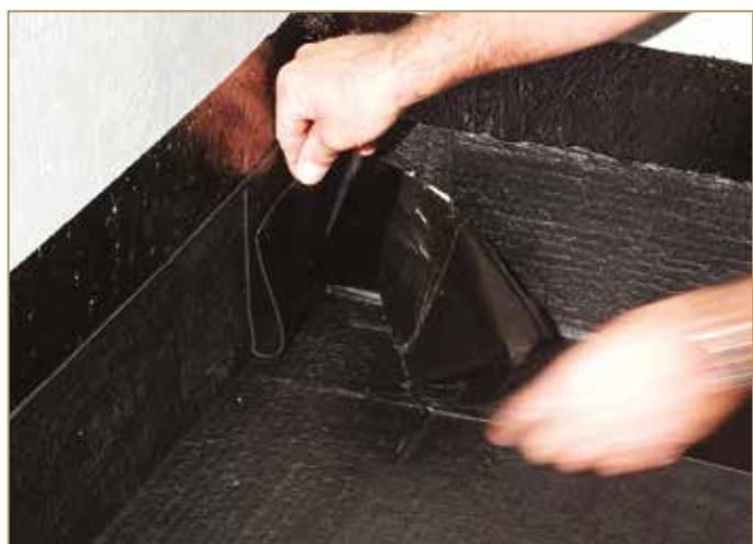
Figure 9.9: Removing the protective film
