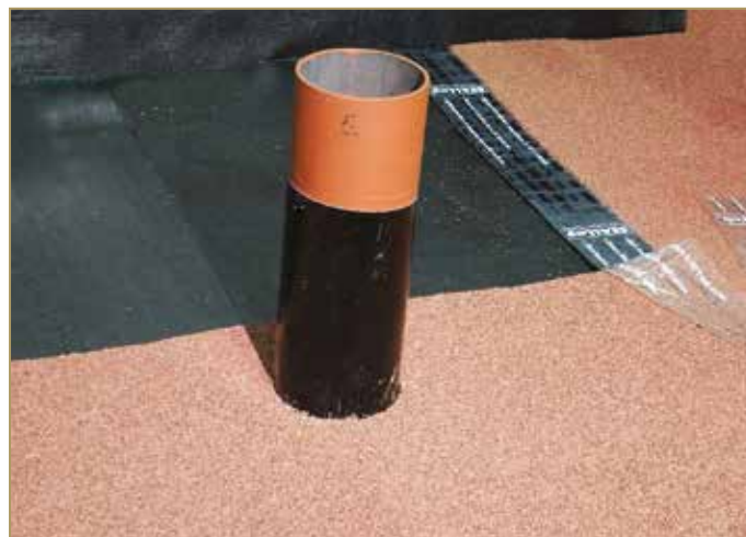
Figure 9.90: Removing the protective film and gluing the second waterproof layer
