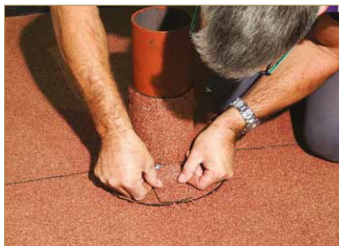
Figure 9.102: Positioning the closing patch
