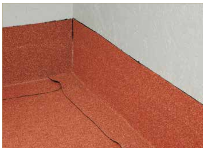
Figure 9.22: Vertical up-turn adhered to the wall
