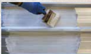
Application on sheet metal
