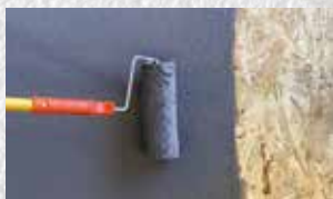
Application on wood
