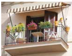
Terraces and balconies
