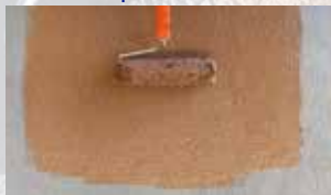
Application on concrete
