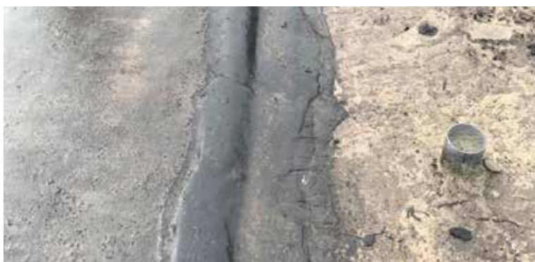
POLYSTRADA SEALANT ensures perfect sealing of cracks and joints, which is one of the most effective measures in terms of road and infrastructure maintenance.
