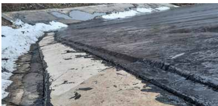
A close-up look of the application of POLYSTRADA SEALANT.
