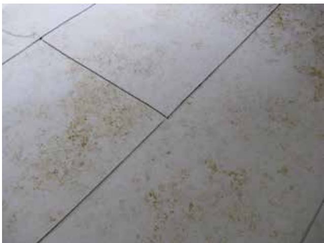
Detail of T-joints.
