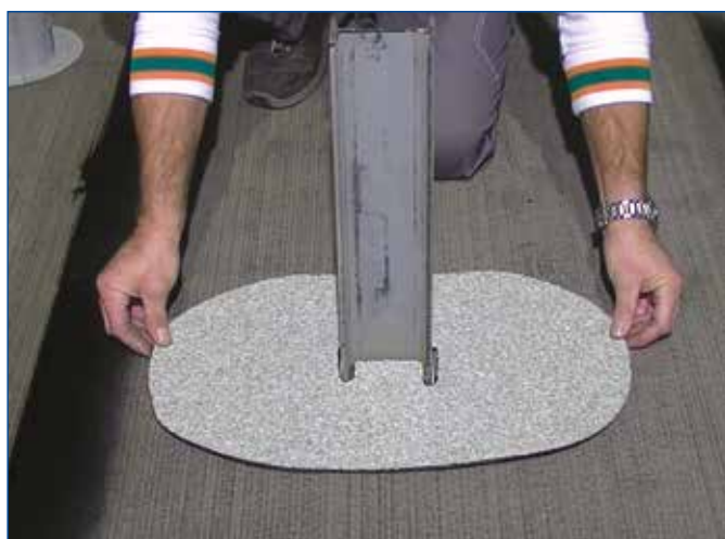
FIGURE 7 - Application of patch of mineral membrane
