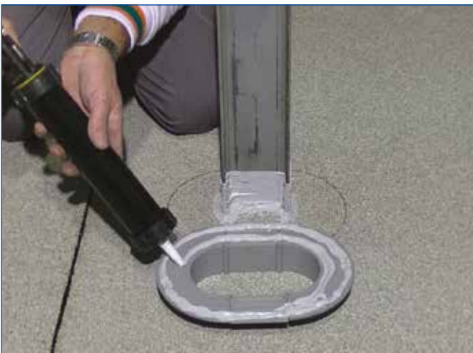
FIGURE 4 - Application of the POLYSEALANT CARTRIDGE adhesive sealant
