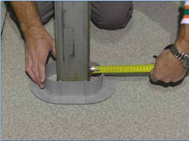
FIGURE 3 - Positioning of the formwork
