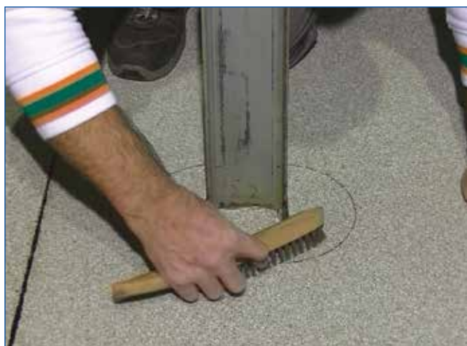
FIGURE 2 - Preparing the surfaces
