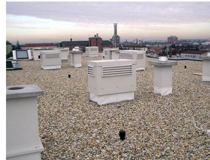
FIGURE 6 SHOWS THE MAPEPLAN INSTALLED ON A ROOF WITH GRAVEL BALLAST
