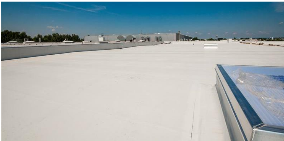
FIGURE 3: MAPEPLAN M ON FULLY EXPOSED ROOF
